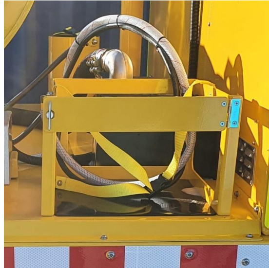
Figure 54: Foam Drum – OS on the Rear Deck.
